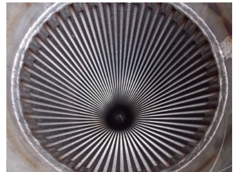
24 in. screen installed
